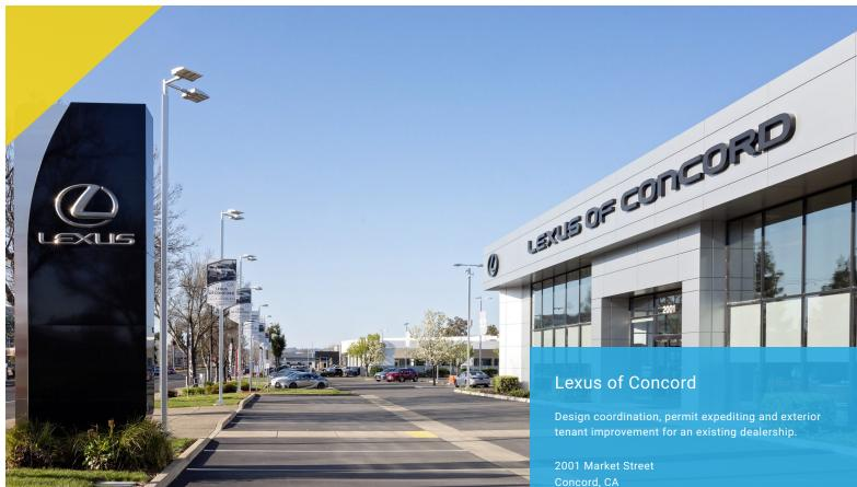
Project scope includes façade improvement, removing the existing stucco building caps at the exterior of two buildings, improving the structure and installing all new metal composite material (MCM) panels. Project phased and occupied.
