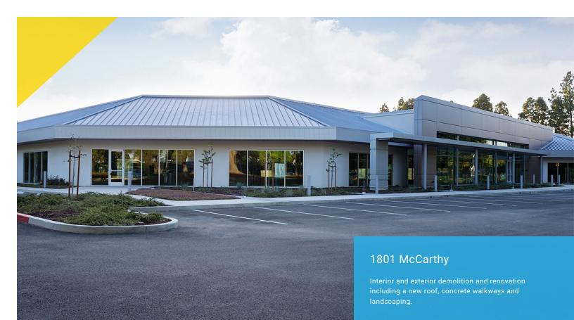
Complete gut of interior and exterior, new roof, new mansard, new feature entrance portal, new paving driveways, concrete walkways and landscaping. The building was additionally prepped to receive 6,000 AMPs of power.
